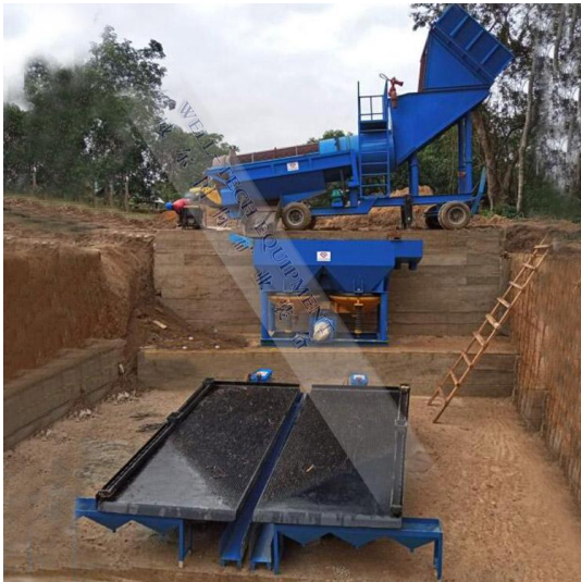
Gold and diamond plant in Liberia
